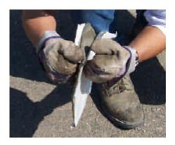
5. Set the Dura-Post™ base on the Butyl Pad, centering it within the edges of the pad. Press on the base to secure it to the pad.
